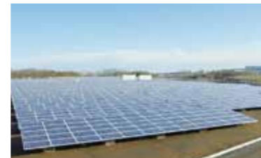
Sanrizuka Solar Power Plant
