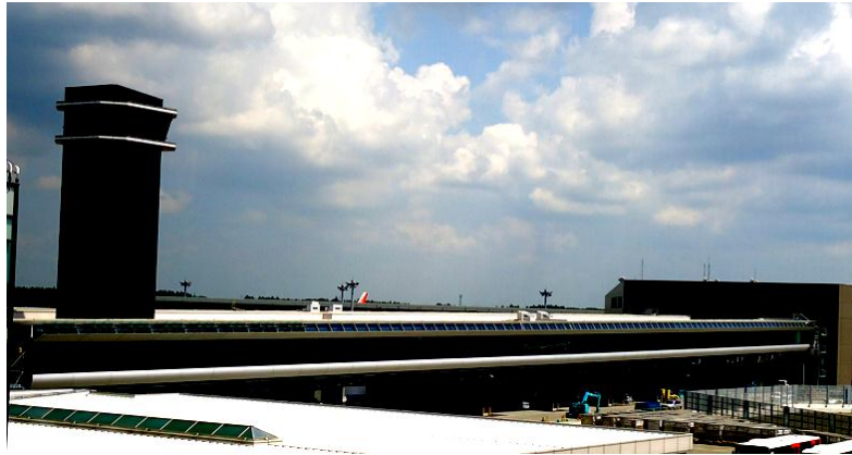
Connecting corridor (external view)
