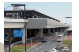
Overhead bridge in front of Terminal 2
