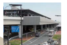
Overhead bridge in front of Terminal 2
