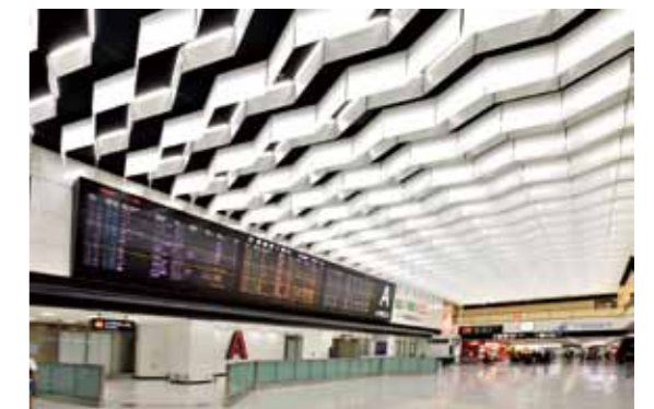
LED lights on the ceiling of international arrival lobby in Passenger Terminal 2
