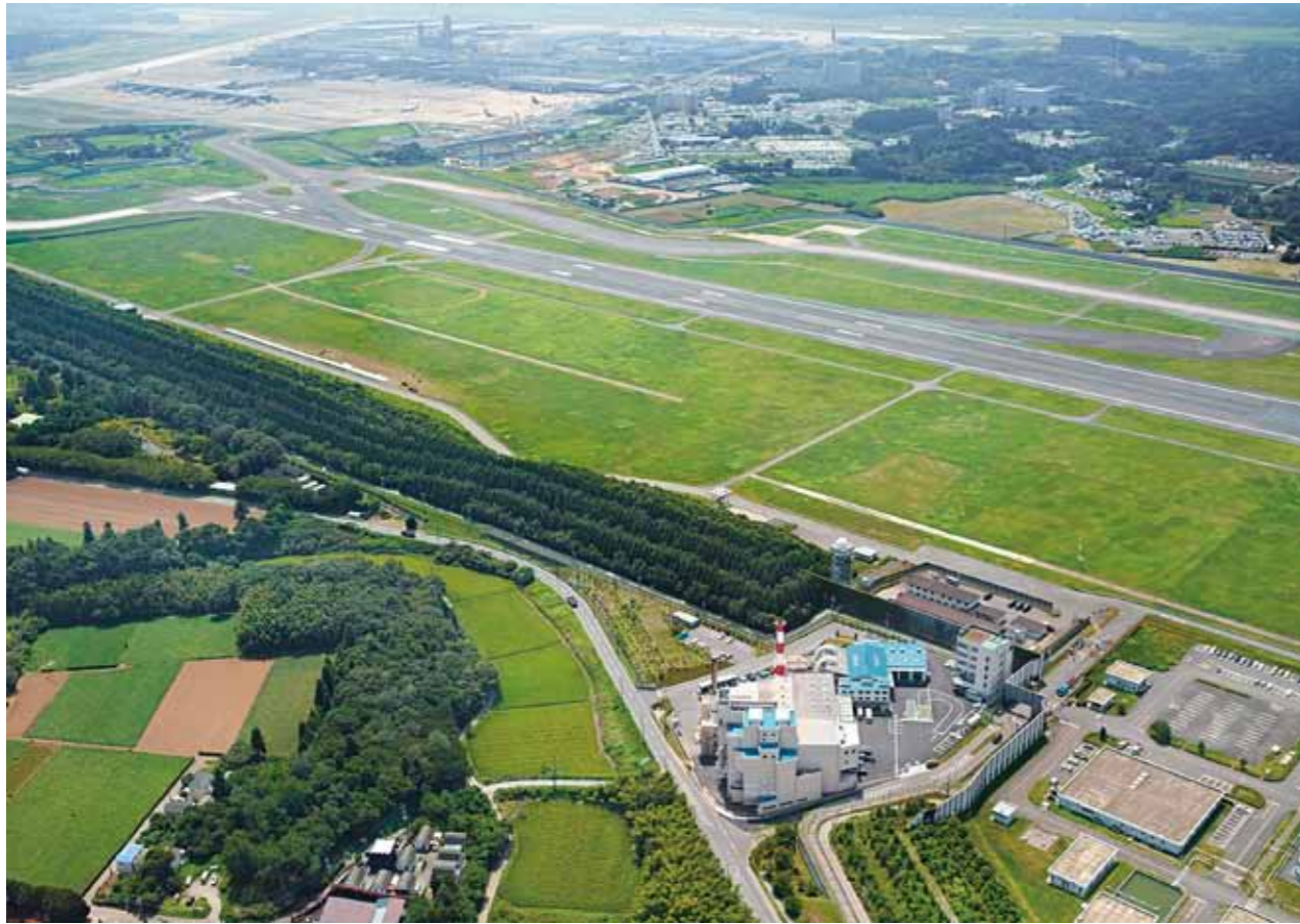
Upper left: Narita International Airport Bottom right: NARIKOH Clean Center, a waste disposal facility
