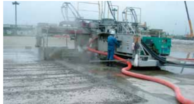
Repair work using the bonded overlay method
