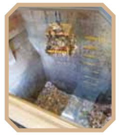
Stirring general waste with a crane to facilitate combustion
