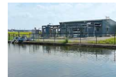
De-icing effluent treatment facility
