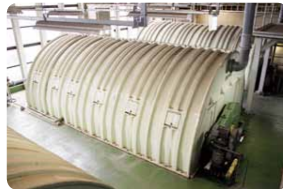
Kitchen wastewater treatment facility
