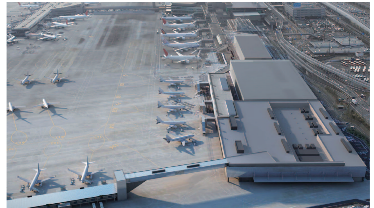
Image of the completed low-cost terminal.
